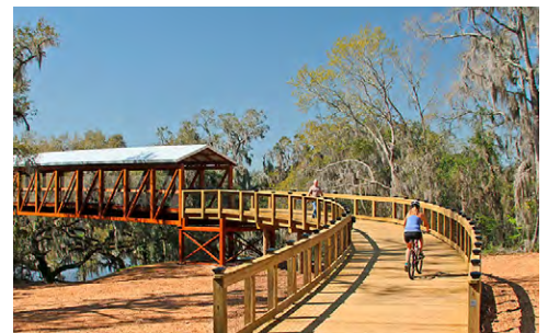
135' Steel Free Span with Timber Deck Lafayette Heritage Park, Tallahassee, FL
