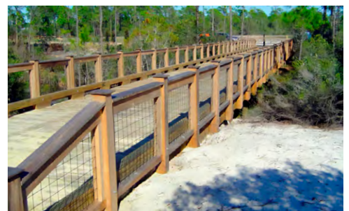
HS10 Bridge, Windmark Beach, Port St Joe, FL
