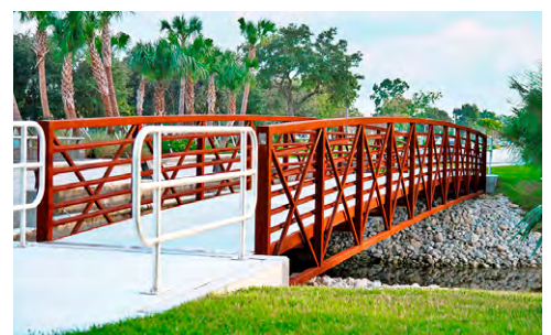
40' Steel Free Span with Concrete Deck Village of Royal Palm Beach, FL
