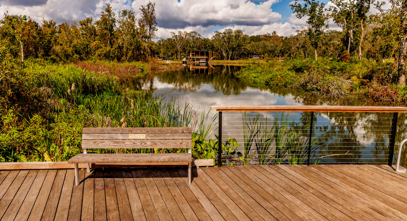
Stainless Steel Cable Rail with Powder Coated Posts Bonnet Springs Park, Lakeland, FL
