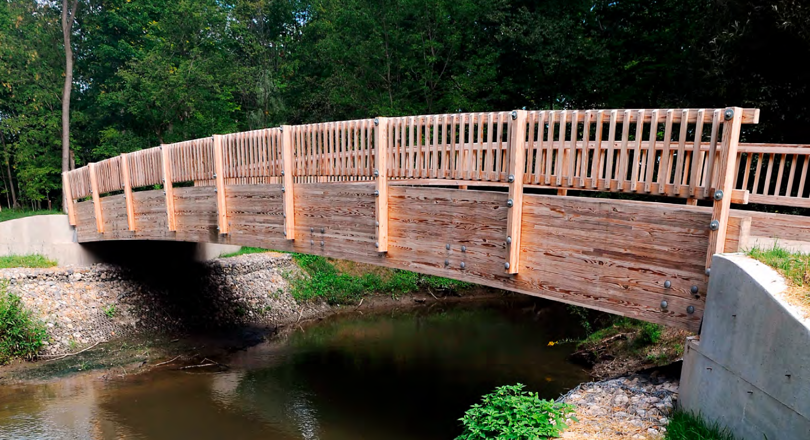
35' Arched Glue-Laminated Timber Free Span Lower Rouge, Canton, MI
