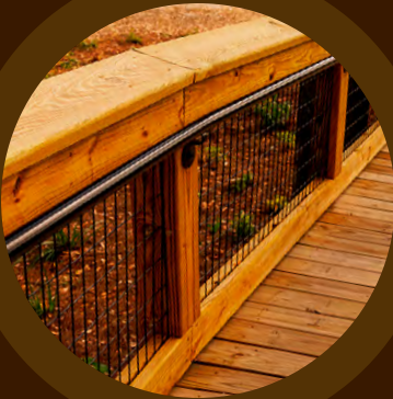
Vinyl Coated Wire Mesh with Wooden Posts and Grab Rails
